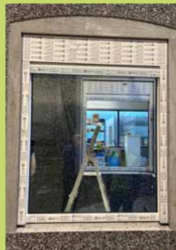
Rullgardinvindu montert i betongelement.
