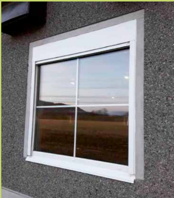
Rullgardinvindu montert i betongelement.
